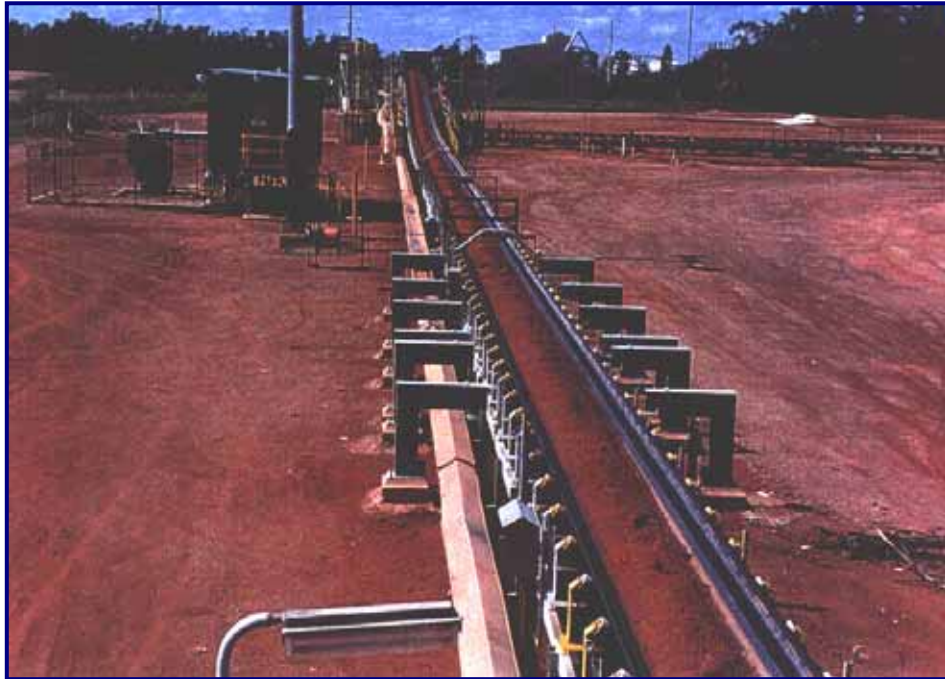
Weipa Dump Station Conveyors
